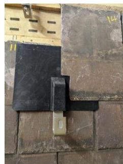
Concrete Tile Flashing
