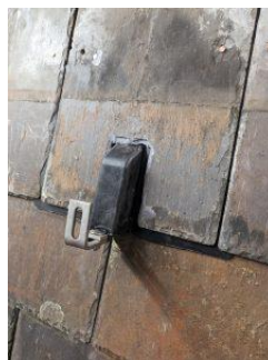
Plain & Slate Tile Flashing
