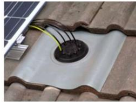
Roof entry lead slate
